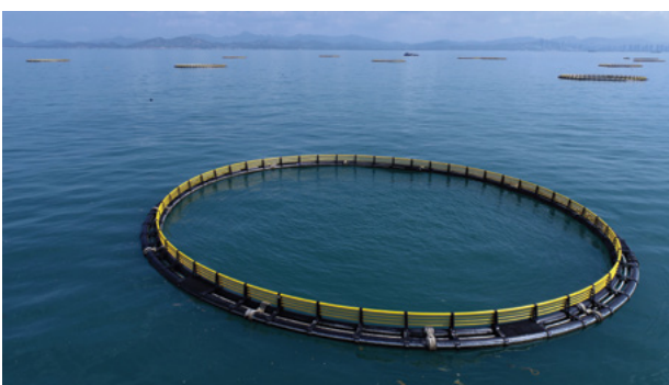
Construction of deep-sea cages in the new culture zones for renting to fishermen associations
